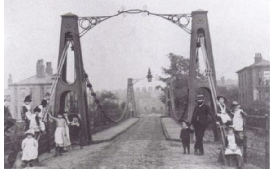
Broughton Suspension Bridge collapsed in 1831
